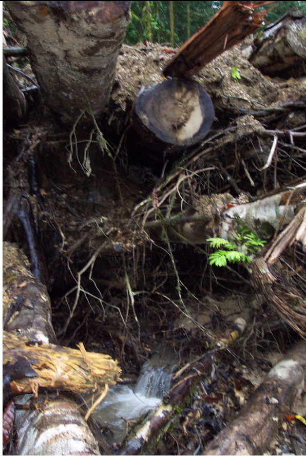
Plate 5 Log Clusters used for water crossing.
