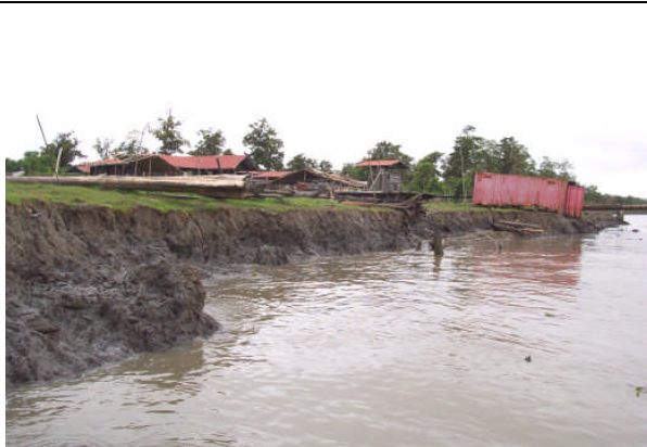
Plate 21 Serious erosion at Station 5.
