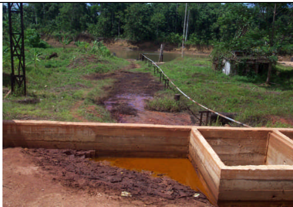
Plate 14 This concrete bund, ( built in November 2003) does not stop fuel oil leaking into the Guavi River.
