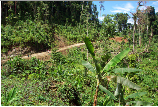
Plate 1. Excessive (> 40 metres) road clearance.
