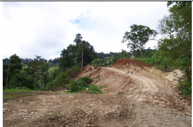
Plate 2. Excessive road clearance due to bad planning.
