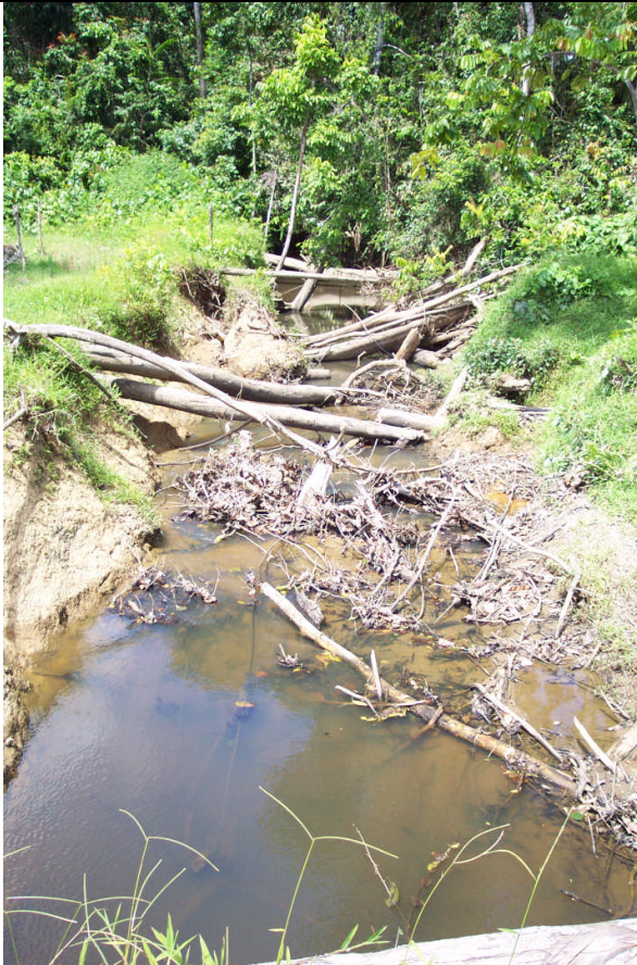
Plate 2 Breaches of Key Standards 1 and 10.
