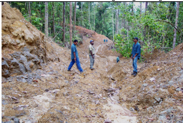
Plate 4 This is a skid track, showing excessive ground disturbance, no water bars, leading to erosion gullies.
